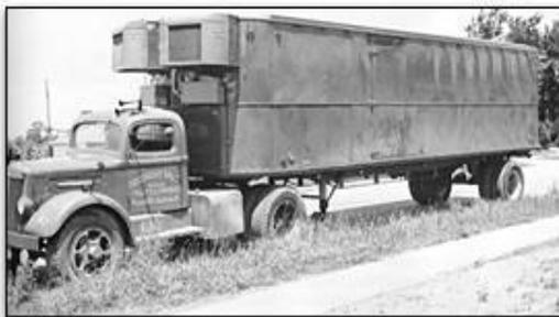
Frederick McKinley Jones decided to invent a machine that would keep the truck cool. In 1949 he received a patent for his air cooling system for trucks. During his lifetime, he invented 40 different types of refrigeration equipment.
